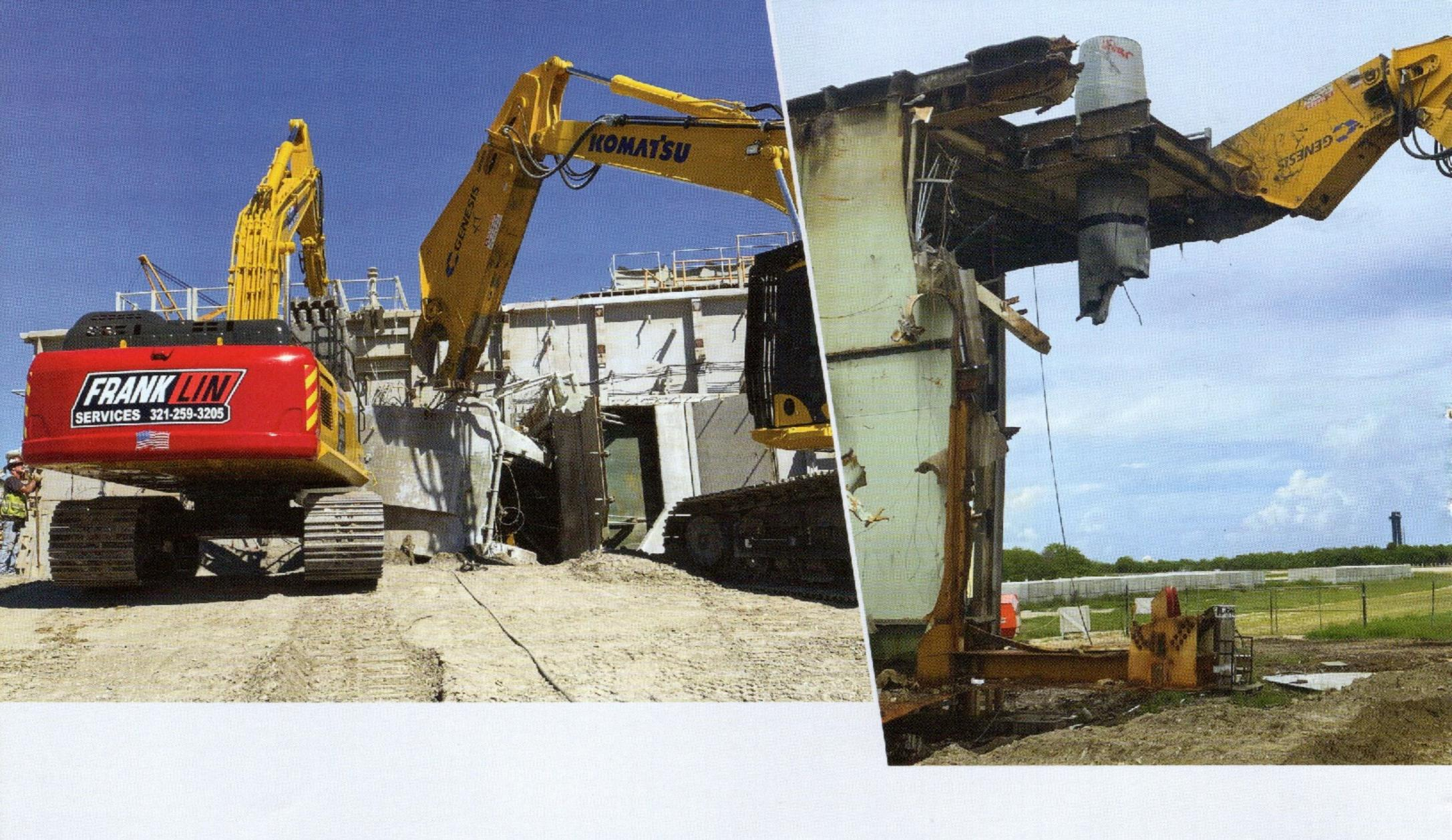
excavators a better position for shearing. With all that in place, we were able to begin the actual demolition of the MLP."
