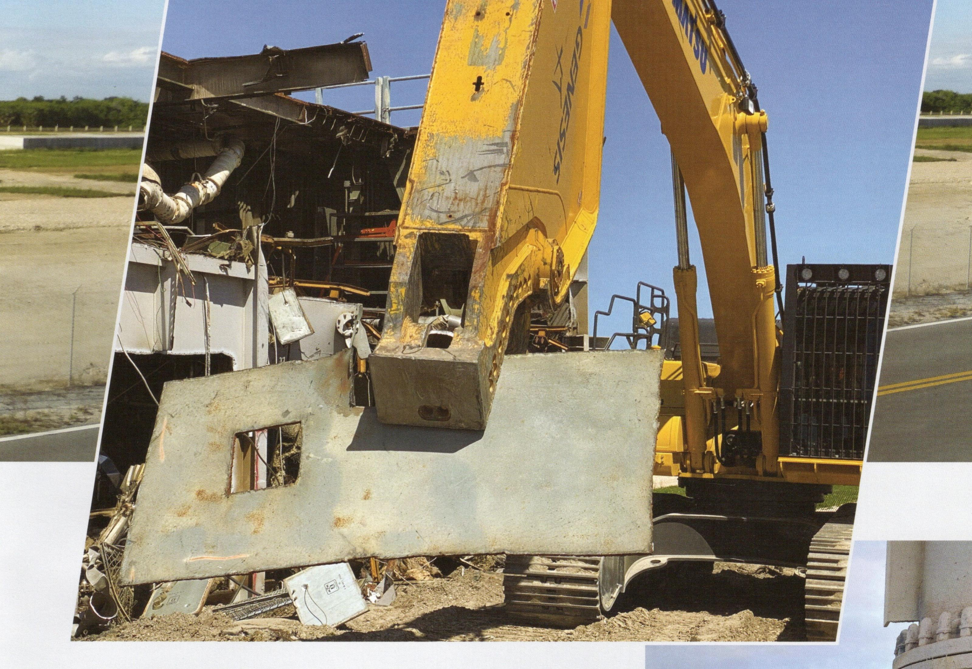
during launch," Charamut says. "That rapid heating/cooling process caused the steel to harden and increased the difficulty factor during dismantling.
