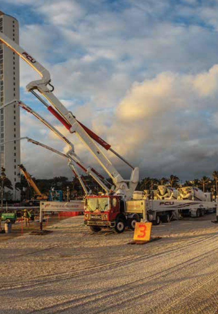
Right: For the foundation mat, a fleet of 100 ready mixed trucks working two shifts fed three Schwing S61 SX truck-mounted concrete pumps and a pair of S46 SX models, pumping more than 14,000 cubic yards of concrete in about 20 hours.
