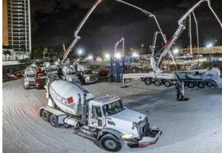
Right: For the foundation mat, a fleet of 100 ready mixed trucks working two shifts fed three Schwing S61 SX truck-mounted concrete pumps and a pair of S46 SX models, pumping more than 14,000 cubic yards of concrete in about 20 hours.
